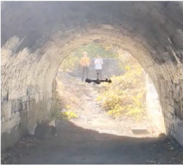
Fig. 12: Integration Test of System in the Miniature Franklin Park Tunnel
